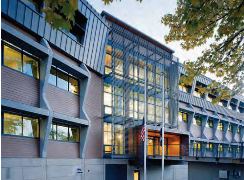
Lewis and Clark State Offices Jefferson City, MO BNIM Architects
