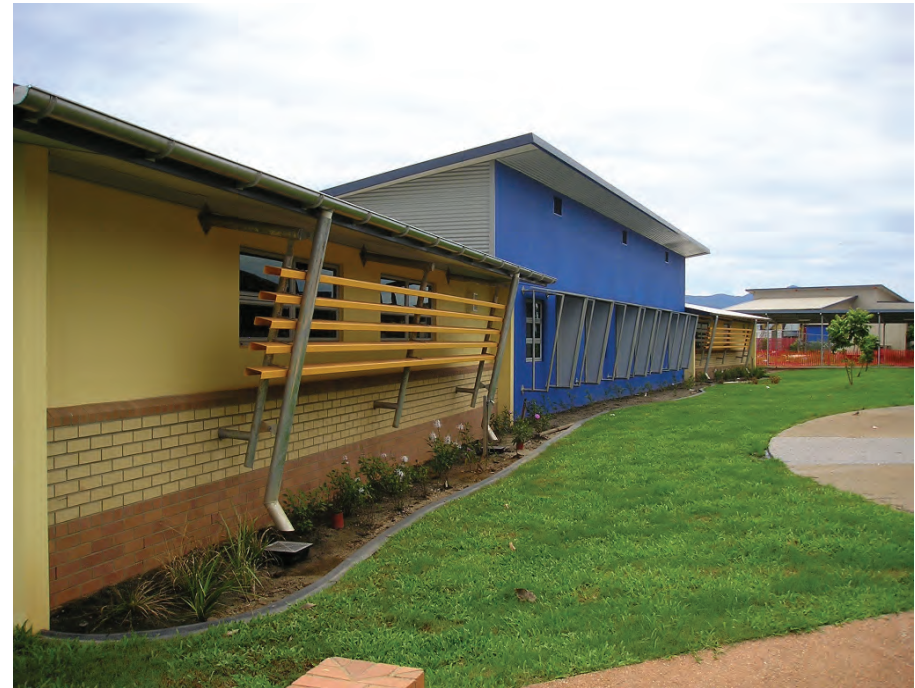
Bentley Park College Cairns, Australia Department of Public Works
